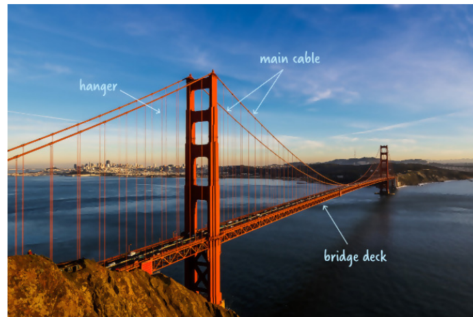
Figure 1: The Golden Gate Bridge
